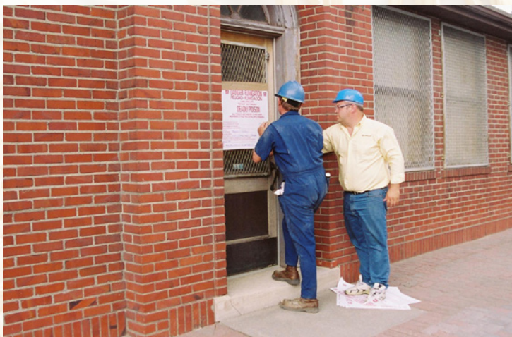
Preparing the Structure
